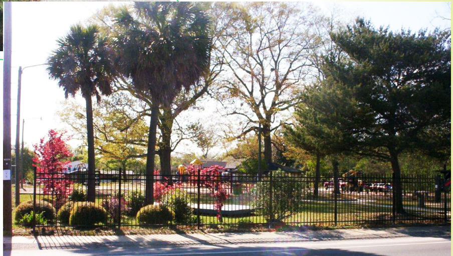
Right: The Pride Park fence after the renovation
