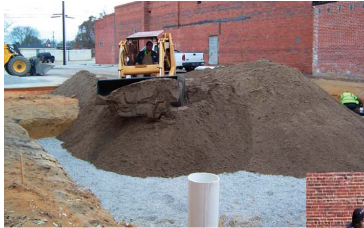
City Rain Garden underway.
